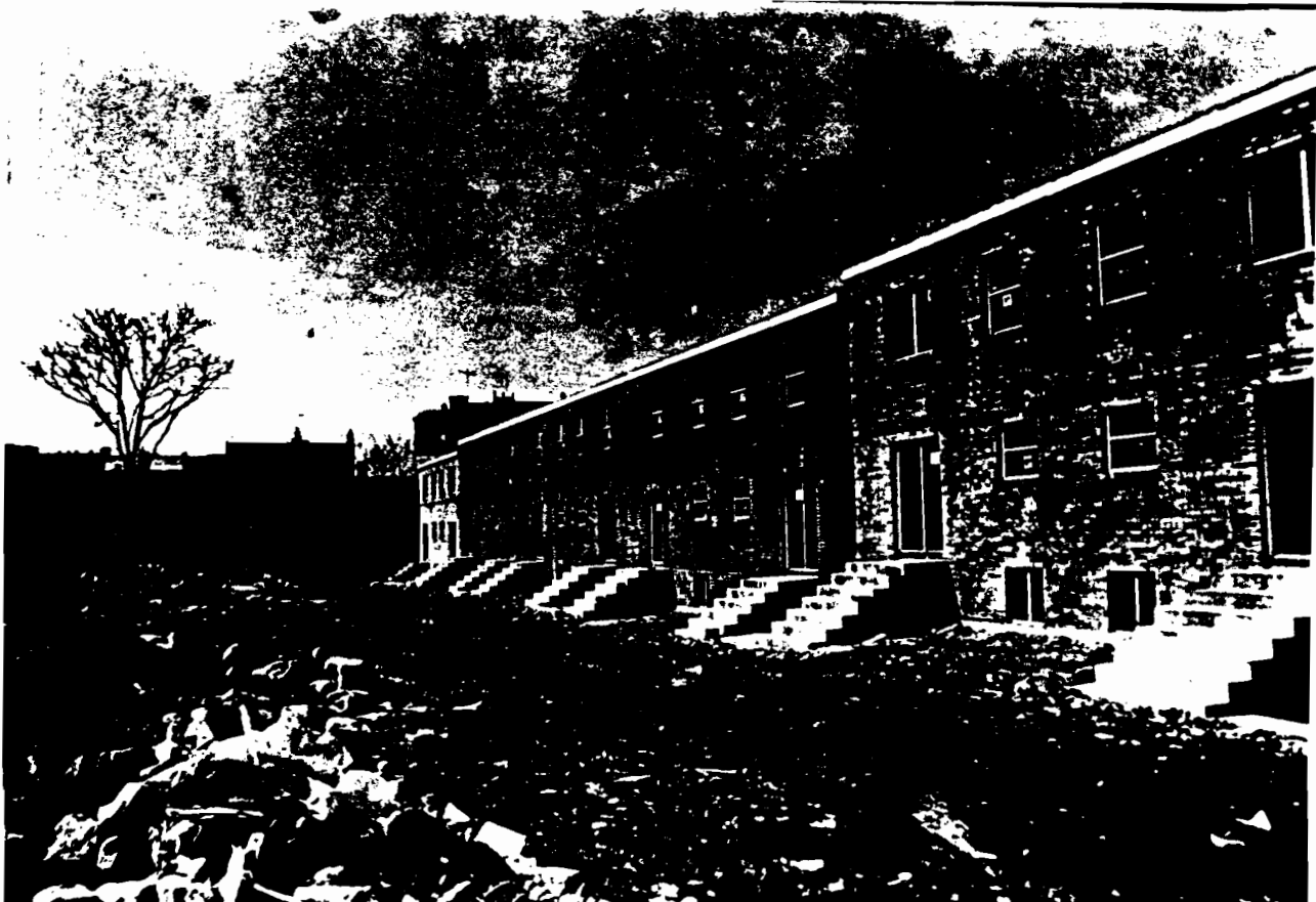
Rear View During Construction. View of Neighborhood in Background
