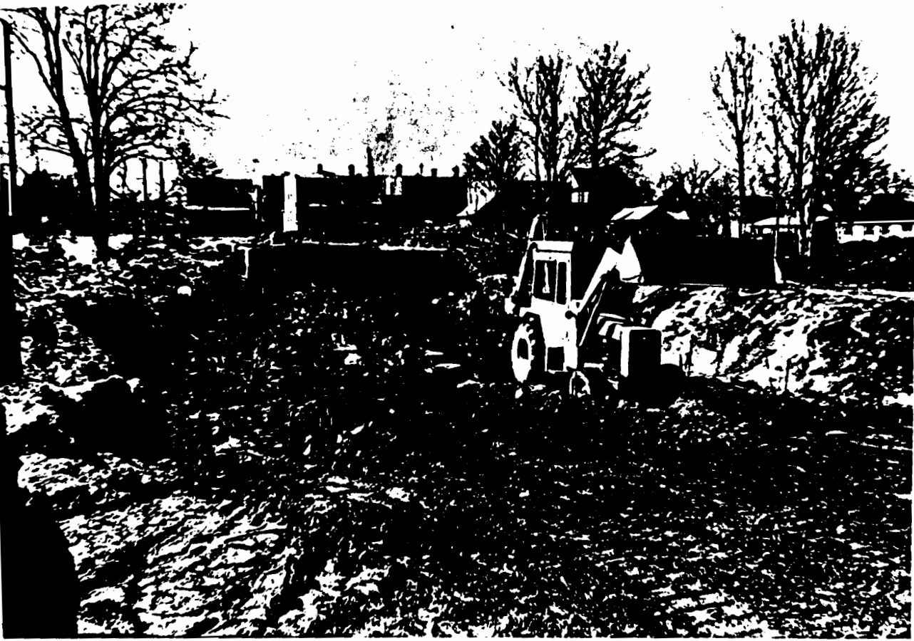
Basement Excavation in Progress and a View of the Surrounding Neighborhood
