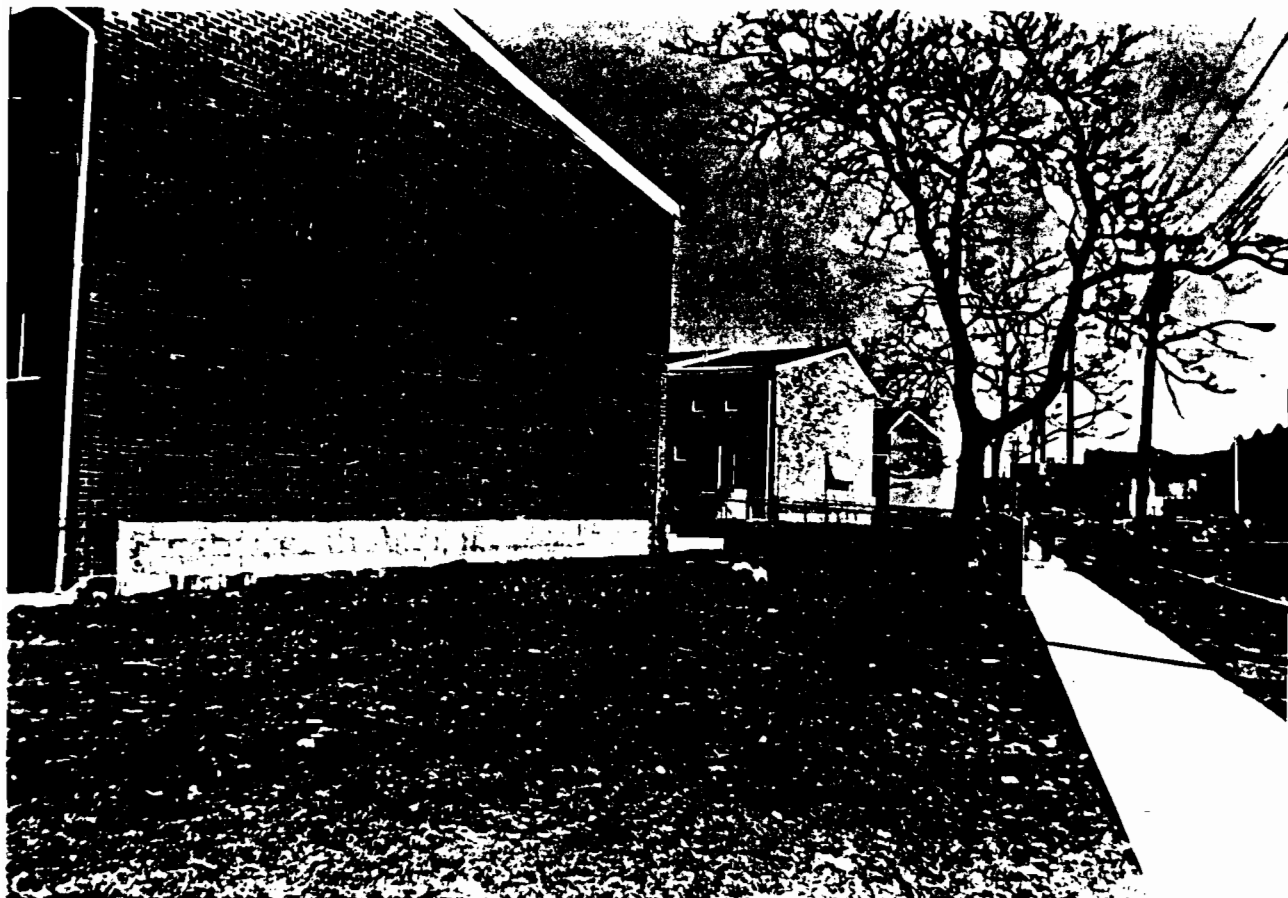
General View as Approaching the Project from the Street
